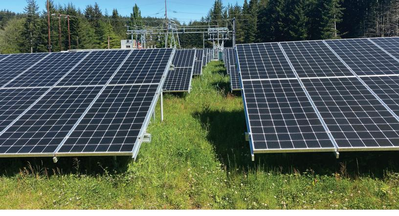
The battery storage project on Decatur is located in the center of the island on 3.6 acres within our main transmission substation and in proximity to our community solar project. The community solar project is a 504 kW DC array that produces approximately 570,000 kWh per year and began producing energy in 2018.
