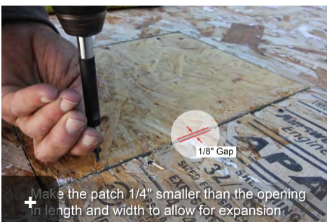
7 Fasten with 2" deck screws
