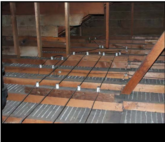
Knob & Tube wiring in an attic.
