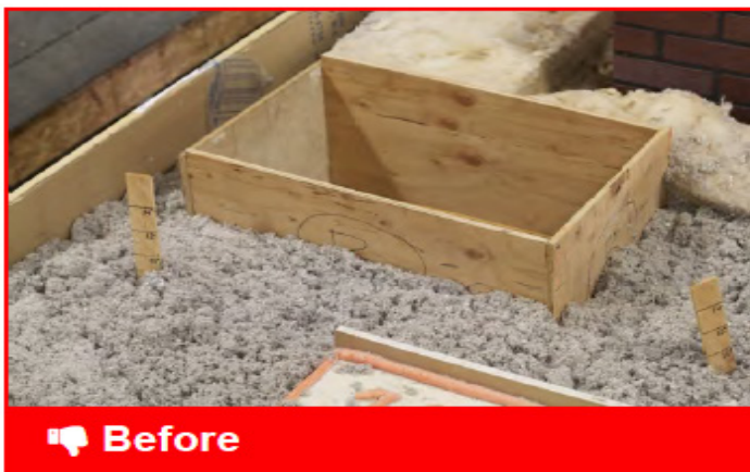
Uninsulated attic hatch
