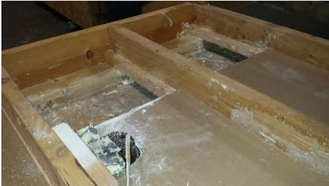
Soffit open to attic
