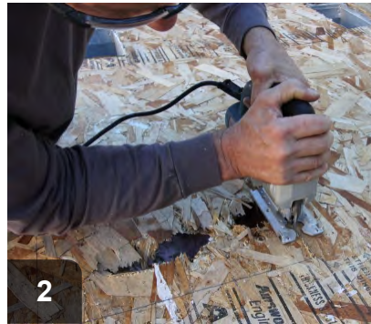
2 Cut out damaged area even with the inside edges of the floor joists
