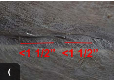
( Staples should be kept tightly together, placed no more than 1 1/2" apart
