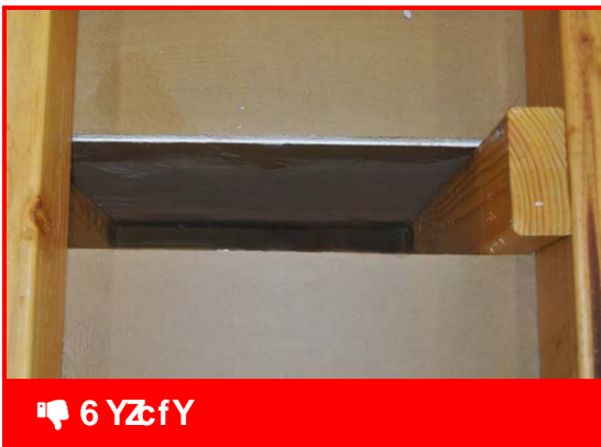
Wall cavities are open to attic
