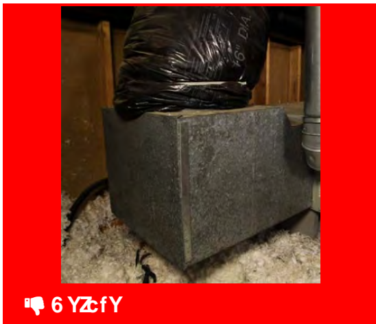
Duct to plenum not sealed
