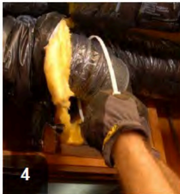
Place panduit strap around the connection.
