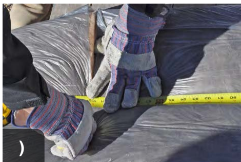
Measure batt to length of cavity with extra for overlap from stuffing tool
