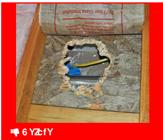
Damage to an older ceiling reveals the new ceiling below
