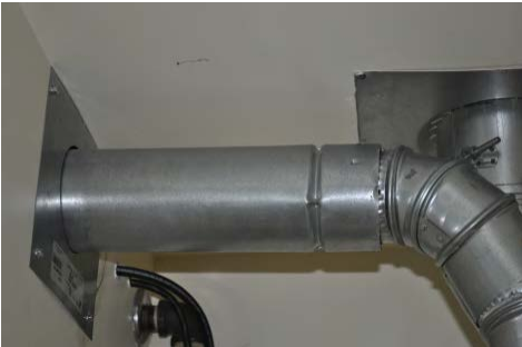
Inspect ventilation systems for inadequate slope
