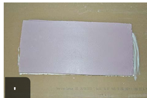
Trim rigid material, such as drywall or XPS, to size and place over sealant
