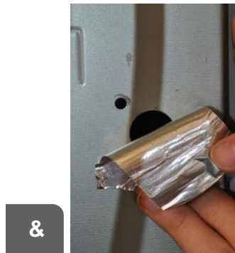
Removable foil tape should be used to seal
