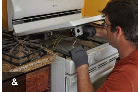
Gas ranges should be cleaned and tuned if improper operation is evident
