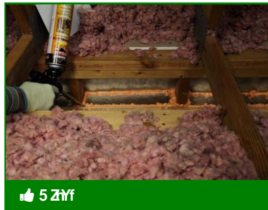
Wall cavities capped and air-sealed in one of a variety of options
