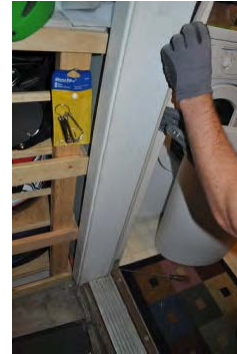
Install weatherstripping into rabbit around door
