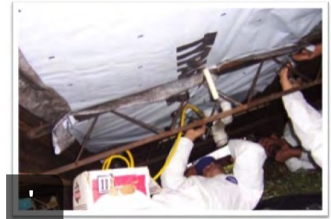
Workers install new material where rodent barrier is missing.
