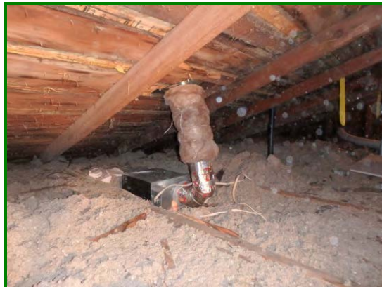
Insulated fan venting prior to addition of loose fill cellulose.
