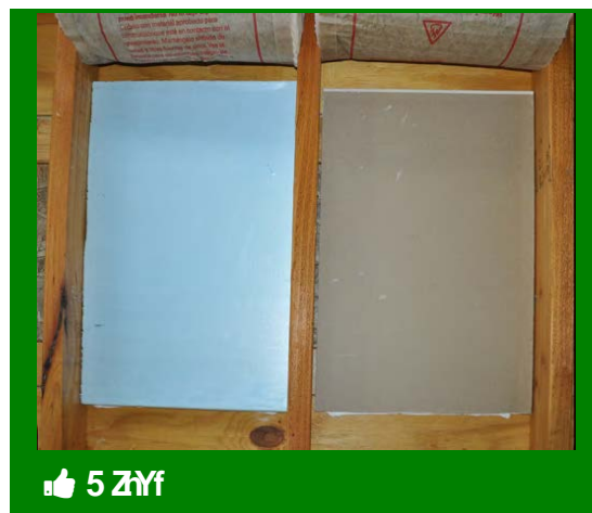
Rigid material sealed in place creates an air barrier
