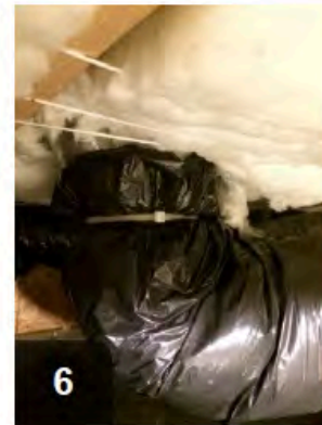
Pull flex duct insulation to cover rigid ducting, then secure outer covering over rigid duct with panduit strap.
