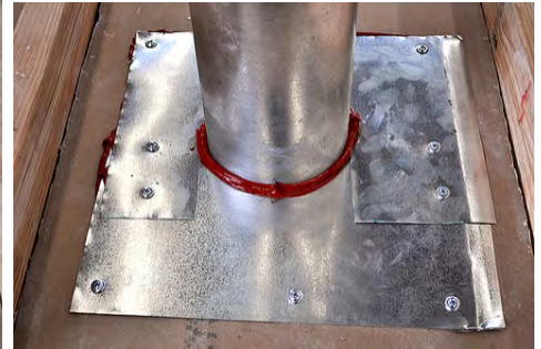
Only construct dam after sealing has been completed properly
