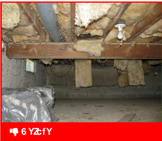
Uncovered crawl space floors can cause moisture damage
