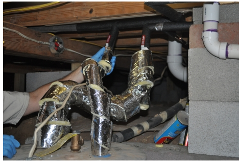
Both hot and cold water pipes should be insulated to R-3 for first 6'
