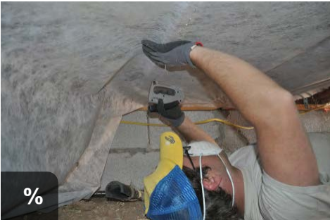
% Secure netting across each joist to create separate cavities
