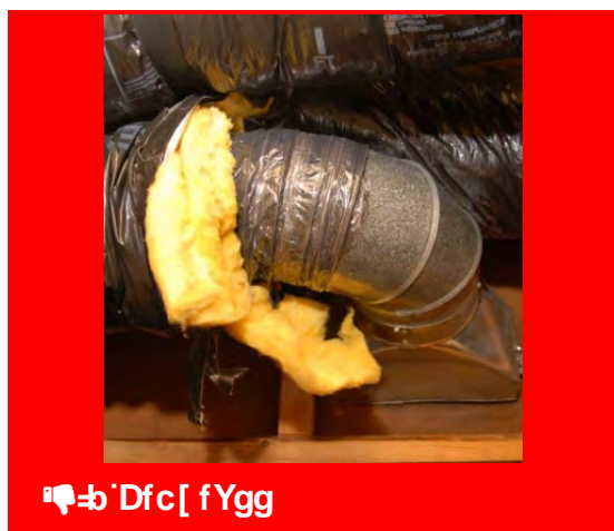
Inner liner of flex duct secured with panduit straps
