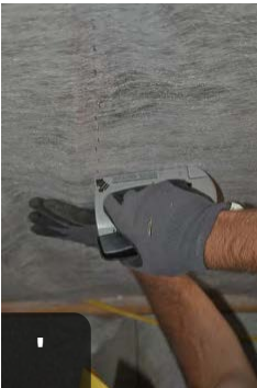
' Keep netting taut while stapling to prevent wrinkles and leakage
