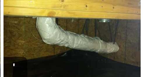
3 Supported and Insulated dryer vent through unconditioned space. Venting slopes downward toward termination.
