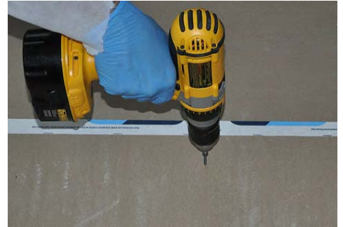
Option 1, Step 3: Secure the rigid material with screws
