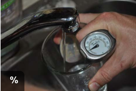
Test temperature of hot water at faucets in house
