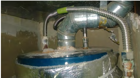
Inspect for missing draft diverter
