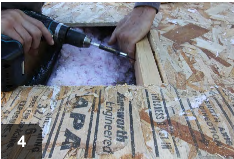
4 Install nailers flat against the joists. Finish by toenailing or screwing 2X4s between the joists
