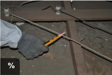
First determine whether K&T wiring is active using an AC voltage detector. The tip glows red for active wiring.
