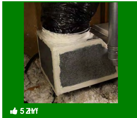
Duct to plenum sealed
