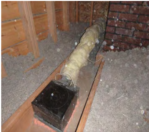
Insulate exhaust fan ducting to R-8 when in unconditioned space.
