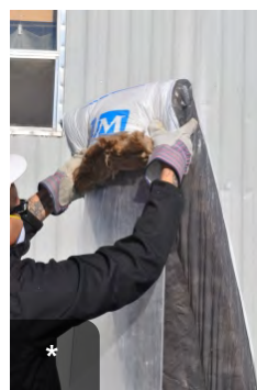
Lap cut batt over bent end of stuffing tool
