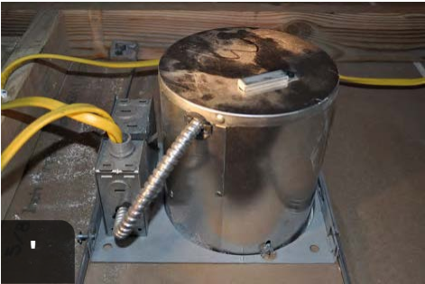
OR non-IC can light can be replaced with IC-rated recessed light
