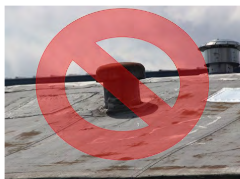
Mushroom vents must be replaced, or removed and sealed.
