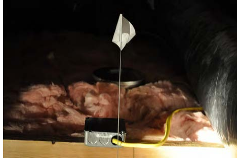
Flag and install covers on electrical junctions
