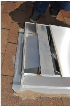
Backdraft damper on roof mounted exhaust fan
