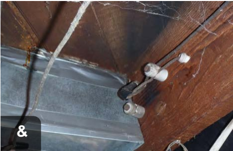
Remember, K&T wiring can be beneath the floor and in wall cavities too.
