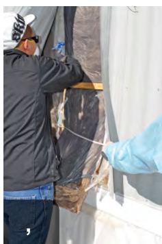
Tuck bottom of batt behind bottom belt rail. If longer than cavity, cut to within 1" longer, roll and tuck into cavity
