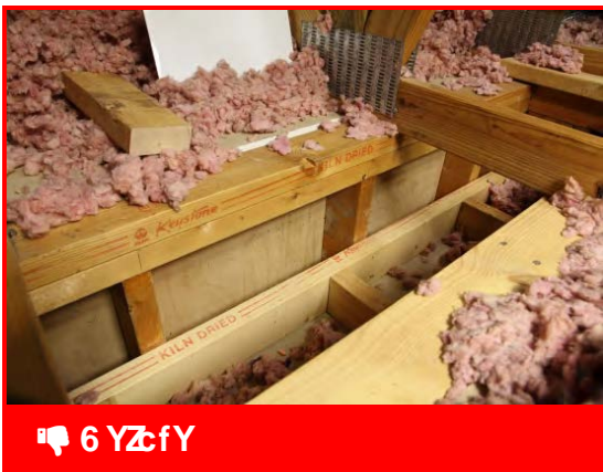
Wall cavities are open to attic and heat transfer due to dropped soffit
