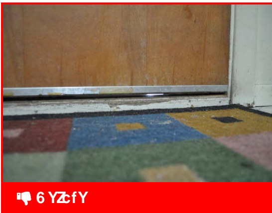
Daylight visible under door to garage indicates leakage
