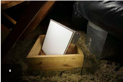
Hatch shall be tight fitting. Install weather strip if needed.
