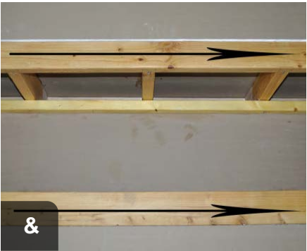
Apply sealant along top plates
