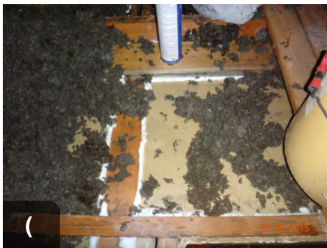
Top plate sealed to ceiling material.
