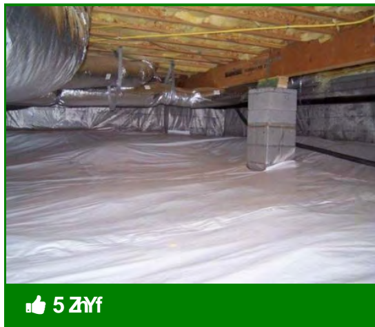
Ground moisture barrier to cover 100% of floor is installed last
