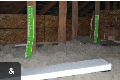
Use depth markers to ensure insulation has reached prescribed R-value
