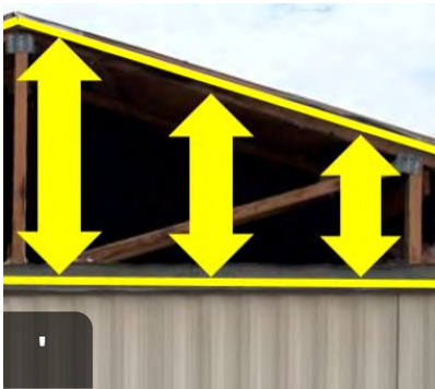
3 If insulation is mounted at both the ceiling and the roof, blow between it.
