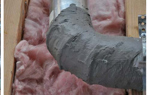
Apply UL 181 mastic to seal joint.
