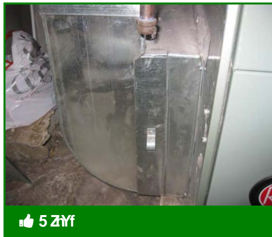
Filter slots should be covered
