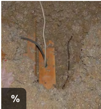
Locate wall tops in attic and look for plumbing and electrical penetrations.
