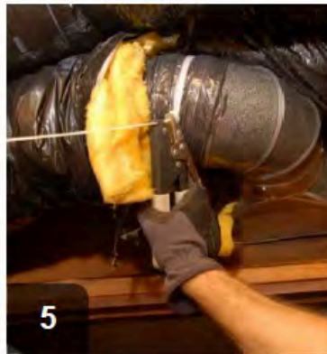
Tighten panduit strap using a tensioning tool.
