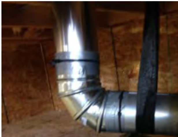
Rigid vent material supported with nylon strapping
