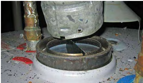
Inspect ventilation systems for disconnected pipes
