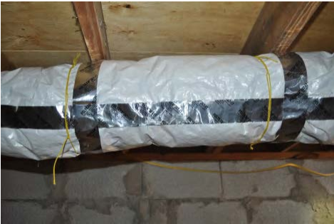
R-8 is the minimum insulation level in unconditioned spaces. Insulation requires a vapor retarder.
