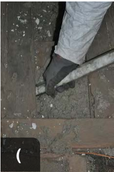
Where flooring cannot be removed, verify insulation is meeting R-value goal
