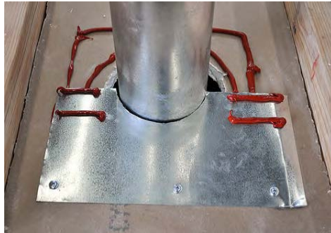
Rigid, non-combustible material should be used to construct seals and dams on flues
