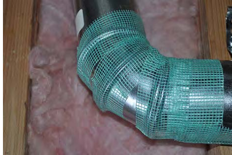
Wrap joint with fiberglass mesh tape.
