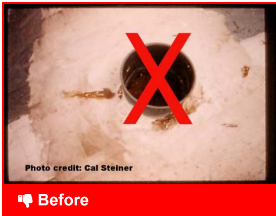
Roof leak, missing cap on vent
