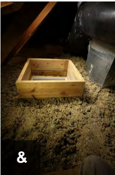
Build dam to hold back attic insulation and hold cover in place tightly
