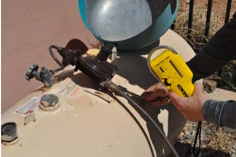
Check all raw fuel lines for leaks
