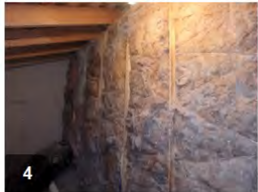
Knee wall insulation is supported by nylon, stapled in a zig zag pattern, 12" on center.
