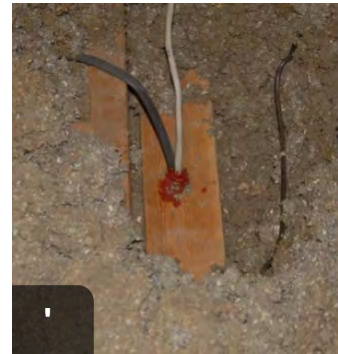
Sealed wall top penetration.
