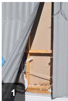
Uninsulated wall cavity can be accessed from exterior of mobile home through paneling
