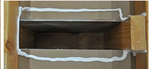
Option 3, Step 1: Apply sealant around opening and on surrounding framing
