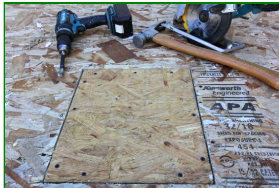
Completed floor repair
