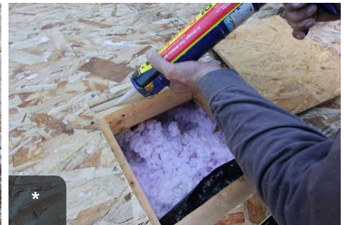
6 Apply subfloor adhesive to nailers
