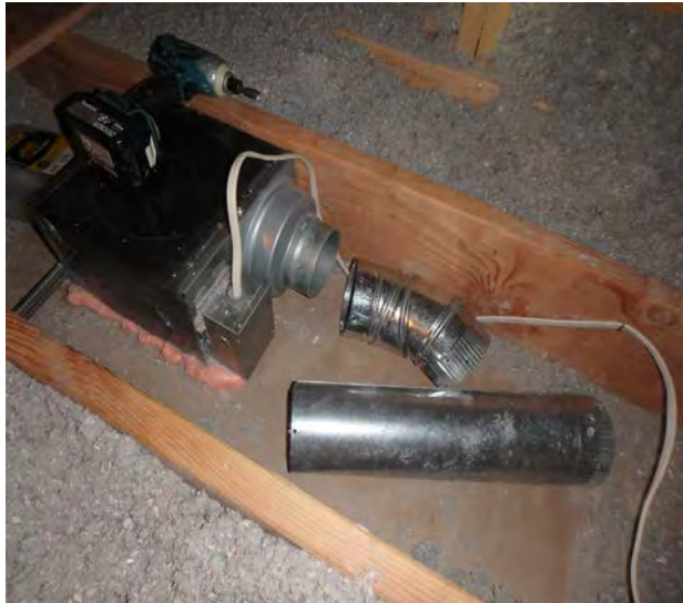
Assemble fan ducting.
