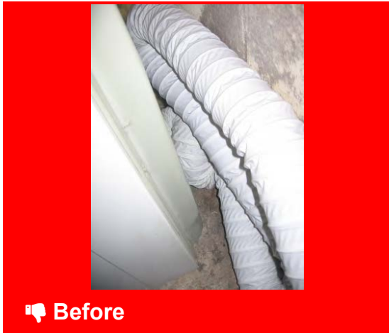
unacceptable dryer venting
