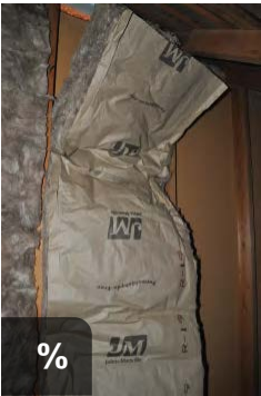
Where existing insulation is improperly installed, fix it
