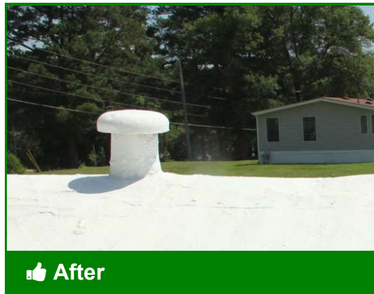
Properly connected and sealed roof vent
