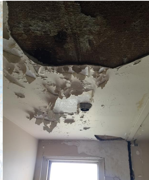
Left: MEP Infrastructure failing and damaging interior plaster walls
