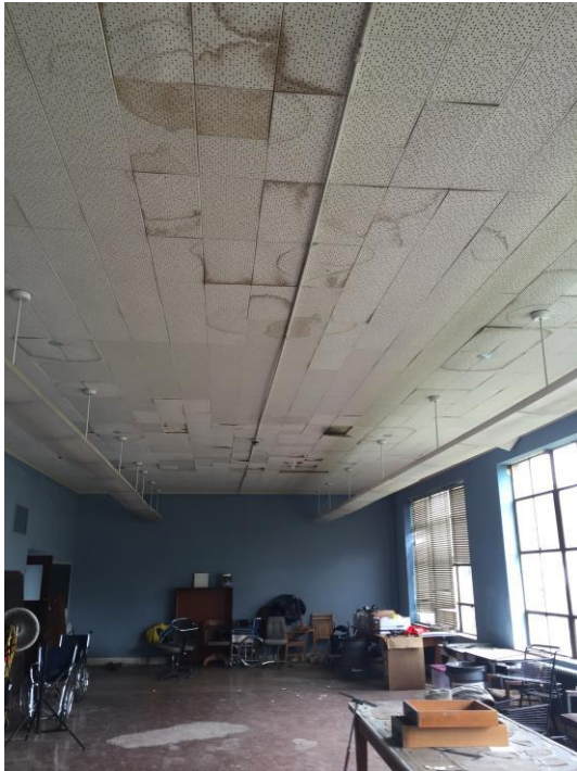
Left: Interior ceiling tile damage and double-hung window disrepair
