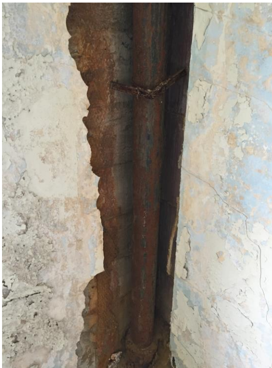
Left: MEP Infrastructure failing and damaging interior plaster walls
