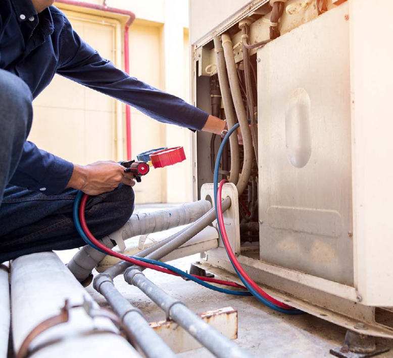
Technician measuring air conditioning equipment.
