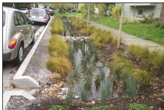
Figure 8 – Typical urban bioswale (Source: American Forests, 2012)
