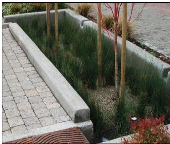
Figure 7 – Typical planter box (Source: Philadelphia Water Department, 2014)
