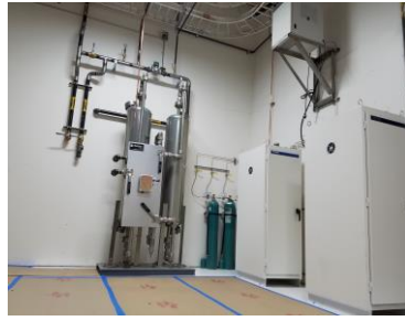
Figure 2: Gas clean up system
