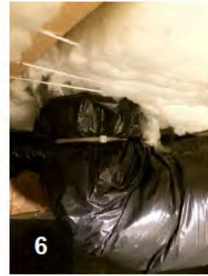
6 Pull flex duct insulation to cover rigid ducting, then secure outer covering over rigid duct with panduit strap.
