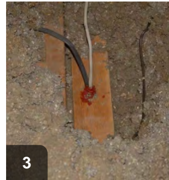
Sealed wall top penetration.
