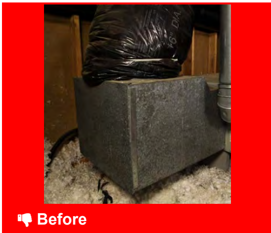
Duct to plenum not sealed
