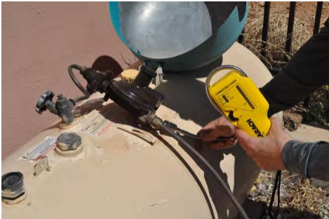
Check all raw fuel lines for leaks
