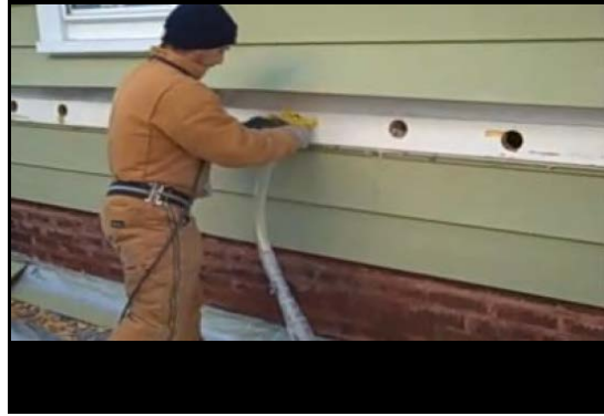
Install insulation to correct density (at least 3.5 pounds per cubic foot for cellulose, or 1.5 pounds for fiberglass)
