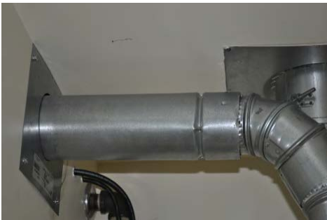
Inspect ventilation systems for inadequate slope
