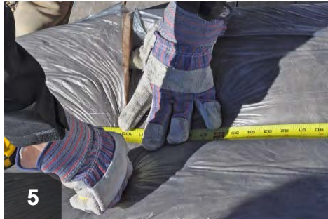
5 Measure batt to length of cavity with extra for overlap from stuffing tool
