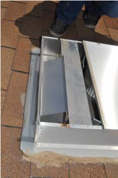
Backdraft damper on roof mounted exhaust fan
