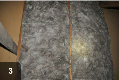
Batts should fill entire volume of knee wall stud bays
