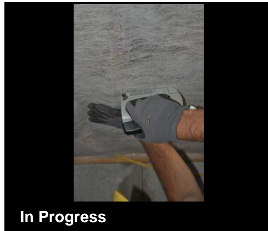
Netting is secured to joists and sills to create cavities for insulation
