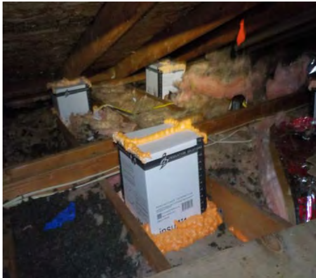
IC rated recessed fixtures can be sealed with fire-rated box assemblies.
