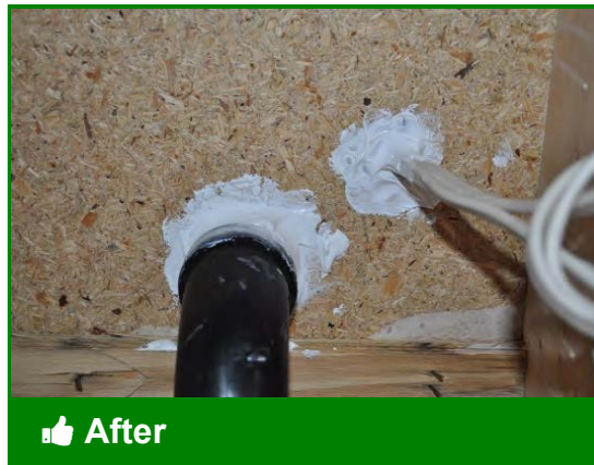
After Sealed penetrations maintain the air barrier
