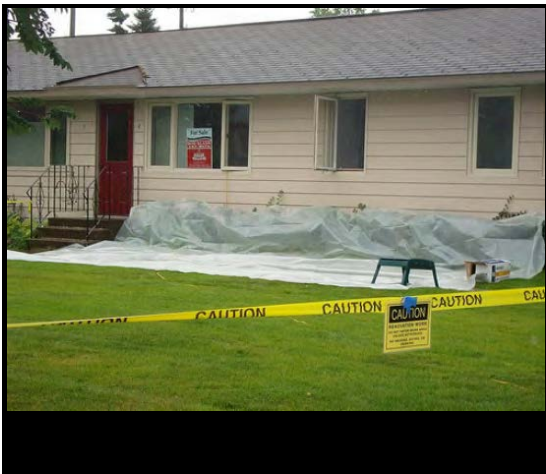
Exterior lead containment elements
