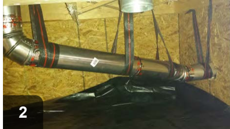
Uninsulated dryer venting in unconditioned space
