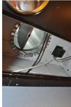
An interior backdraft damper can also be installed for good measure
