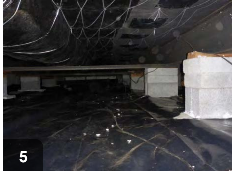
Pin up sagging belly material to prevent installing excessive amounts of insulation material.
