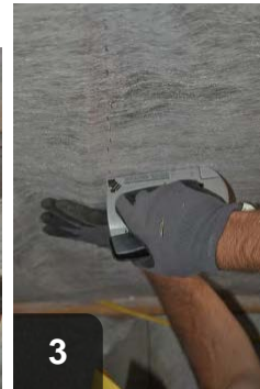
3 Keep netting taut while stapling to prevent wrinkles and leakage
