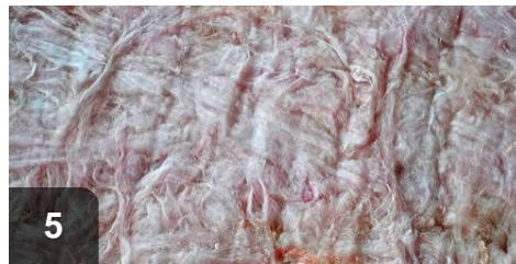
5 Insulate over now-capped soffit
