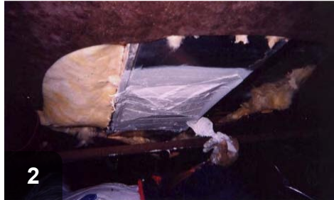
Mobile home duct systems (plenum, trunk terminations) should be sealed from below prior to patching the belly.
