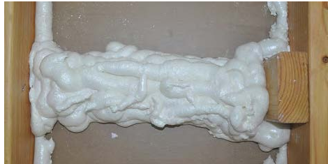
Option 2: Bridge cavities with spray foam
