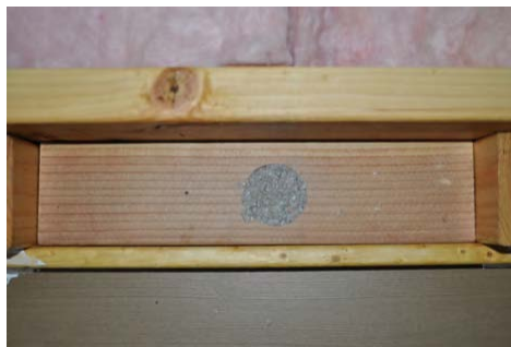
Option 3: Dense pack cavity through fastened wood cap
