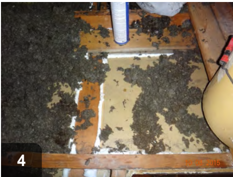
Top plate sealed to ceiling material.
