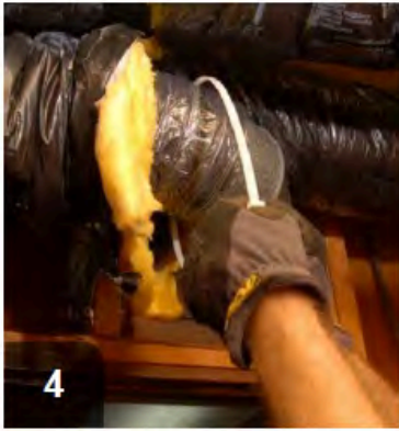
4 Place panduit strap around the connection.
