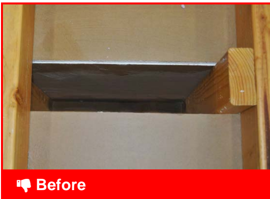
Wall cavities are open to attic
