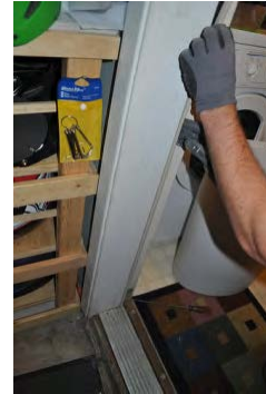
Install weatherstripping into rabbit around door
