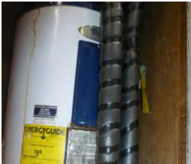
Insulate the first 6 feet of both cold-water and hot-water outlet pipes beginning at the water heater tank
