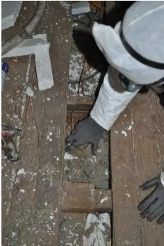
Check cavity for electrical junctions and penetrations
