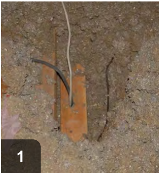
Locate wall tops in attic and look for plumbing and electrical penetrations.
