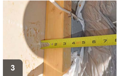
3 Measure depth of cavity
