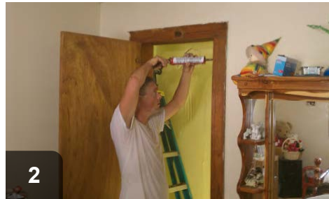
2 Foam, caulk, and seal leaks between halves of double wide manufactured homes
