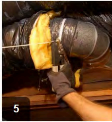
5 Tighten panduit strap using a tensioning tool.
