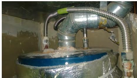
Inspect for missing draft diverter
