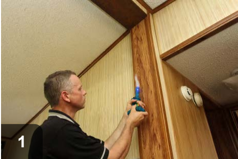
1 Identify leaks in marriage line using a blower door and smoke
