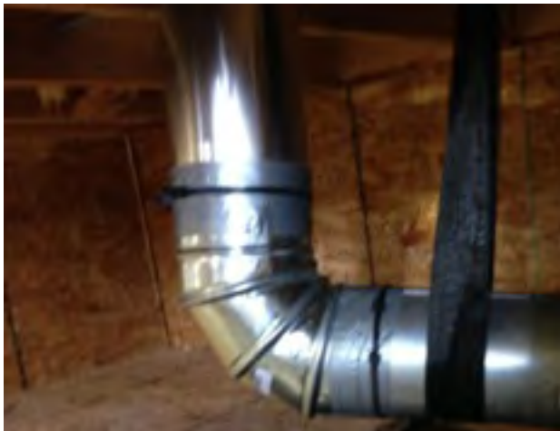
Rigid vent material supported with nylon strapping
