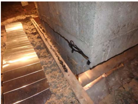
Rigid, non-combustible material should be used to construct seals and dams on chimneys
