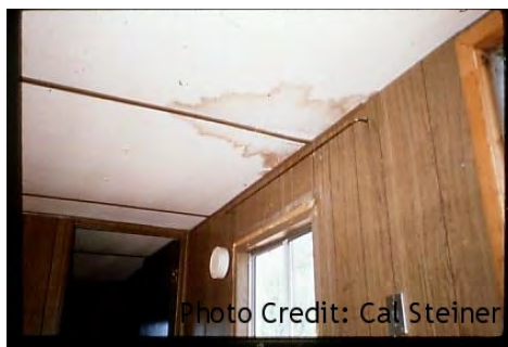
Inspect ceiling for weakness, leaks, clearance to combustibles, loose panels, and penetrations.
