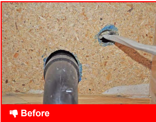
Before Gaps around penetrations can cause air leakage and negate insulation
