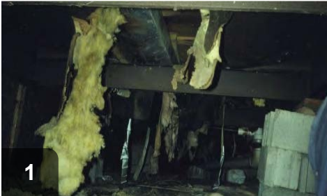
Belly damage: rodent barrier and insulation are damaged, revealing a main supply duct known as a trunk.
