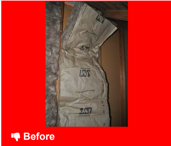
Knee wall with batts improperly installed and missing from stud bays
