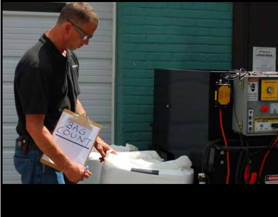
Make accurate count of insulation bags to be installed
