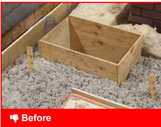
Uninsulated attic hatch
