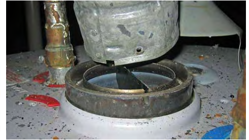
Inspect ventilation systems for disconnected pipes
