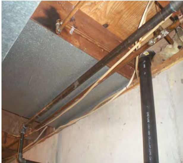
Pan joist return ducting is often leaky, creating depressurization in the zone.
