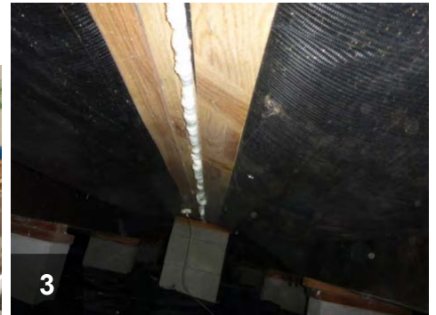
3 Foam sealant has been installed to air seal the floor plane marriage line, accessed from below.
