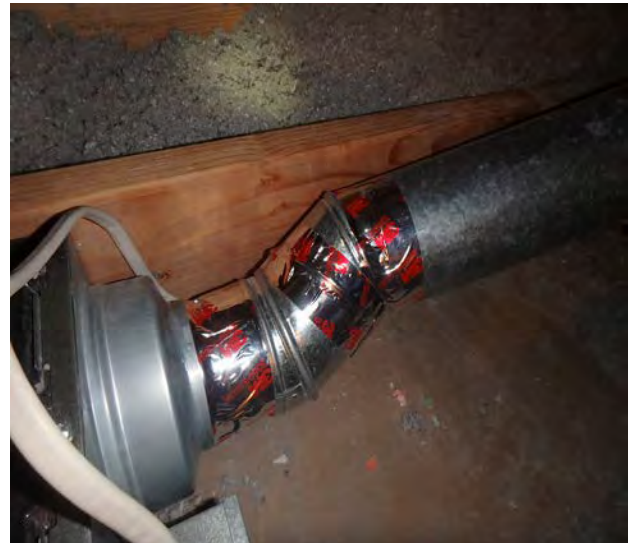
Seal exhaust fan duct seams with mastic or UL181 tape.
