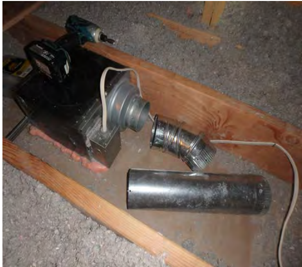
Assemble fan ducting.
