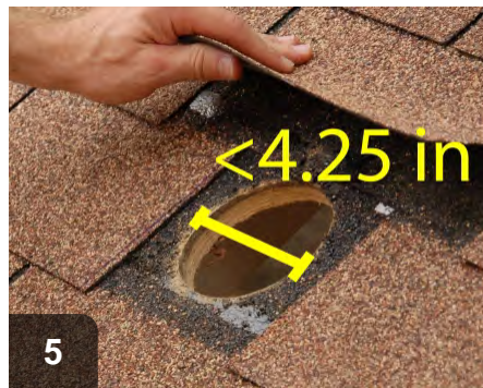
5 Verify hole size is correct before installation
