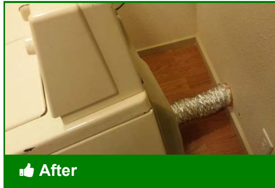
Proper vent material and connection to collar at wall
