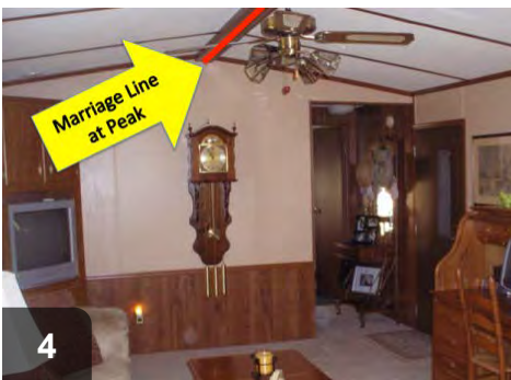
4 Marriage line air sealing of the ceiling plane is accessed from inside the home.
