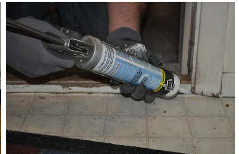
Caulk along threshold to minimize water and contaminant infiltration
