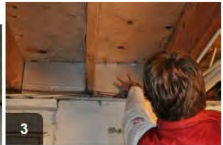
3 Pressure fit rigid insulation into
