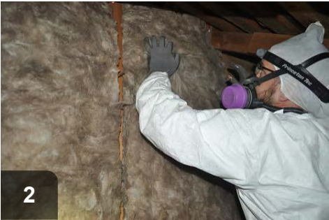
Kraft-face should go to "warm in winter" side and batt should fill bay
