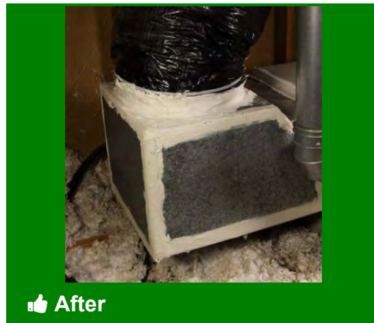
Duct to plenum sealed
