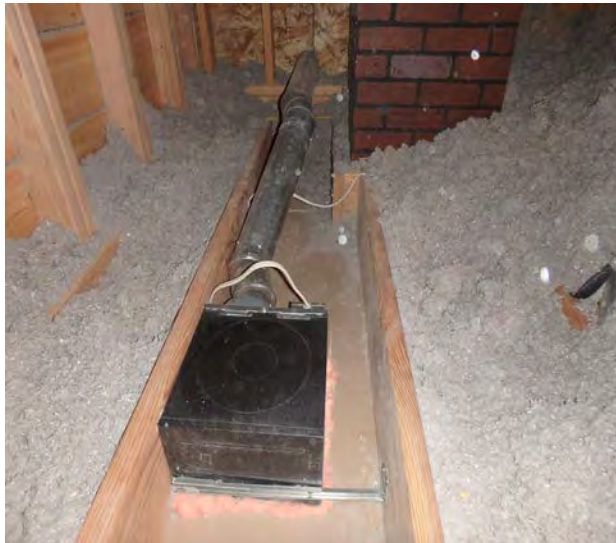
Exhaust fan ducted through vertical surface, still needs to be sealed, insulated, and supported if applicable.
