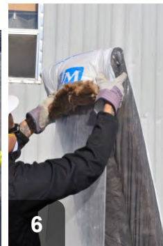
6 Lap cut batt over bent end of stuffing tool
