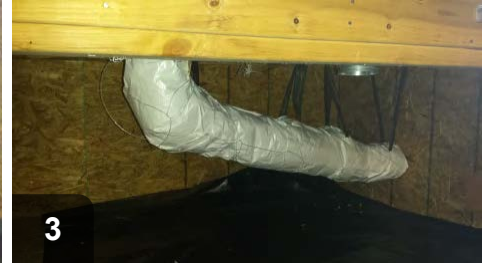
Supported and Insulated dryer vent through unconditioned space. Venting slopes downward toward termination.
