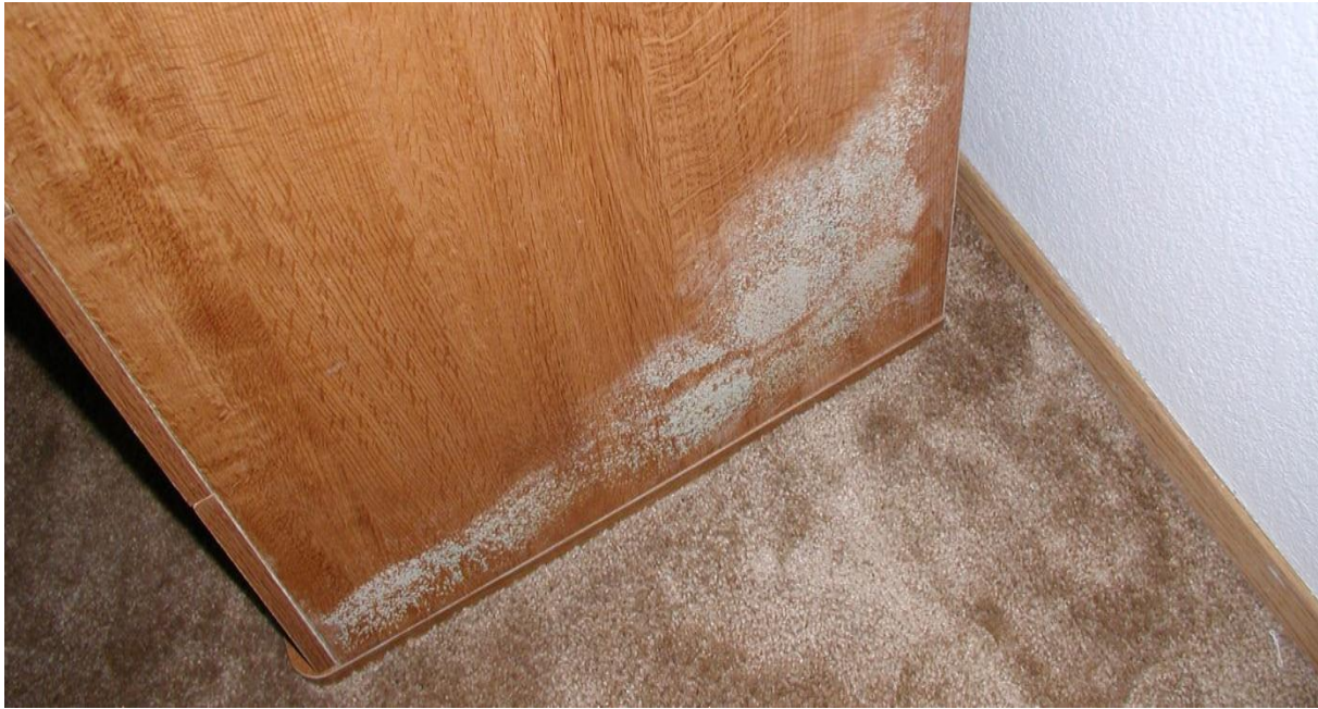
Figure 3. Mold growth caused by condensation on the cool cabinet placed against an exterior wall in a rental unit. The excessive indoor relative humidity (regularly exceeding 60%) was the culprit. This surface can be cleaned with soapy water.
