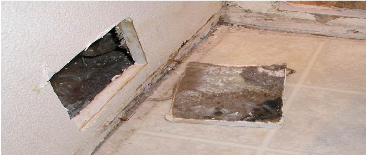
Figure 12. Saturated wallboard must be aggressively dried or mold WILL grow, often on the hidden paper backside of the wallboard in the wall cavity. This moldy wallboard should be carefully abated using a negative pressure enclosure and respiratory protection for workers.
