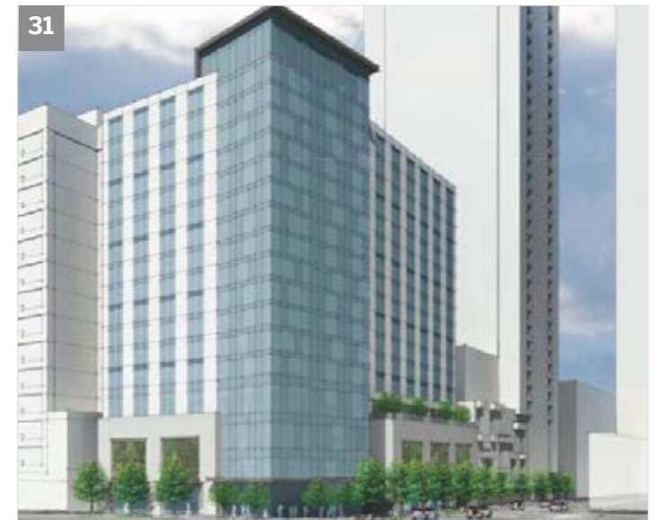
31 924 HOWELL STREET Hotel Under Construction: DPD #3017451
