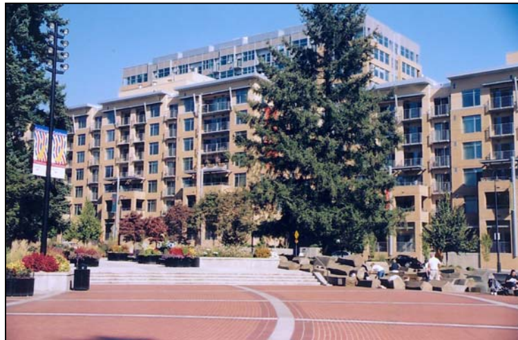
Affordable housing units are being constructed as Vancouver revamps its downtown.
