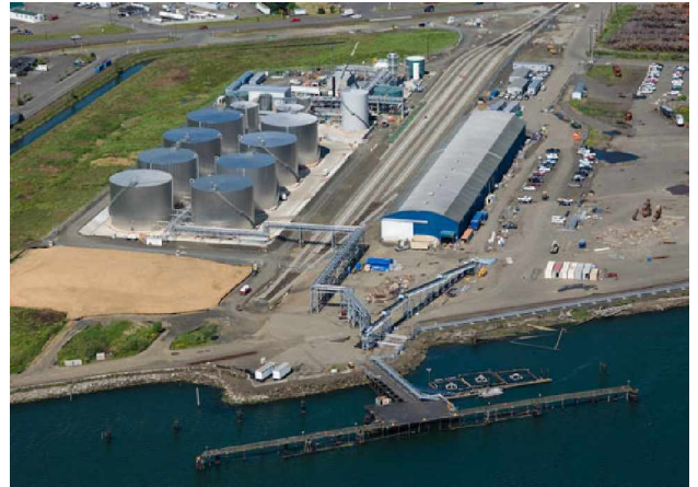
Port of Grays Harbor Terminal 1
