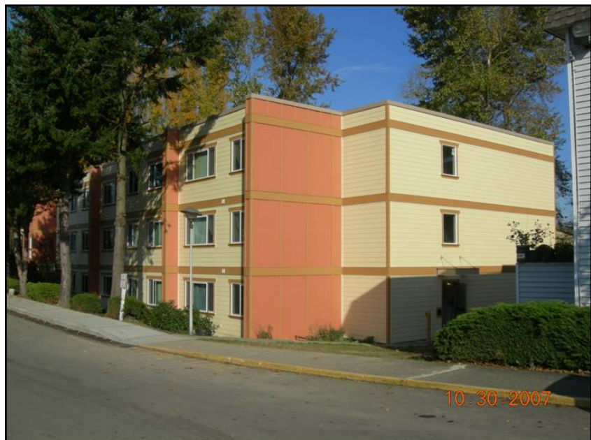
KCHA's Riverton project — after. Cleaner, safer, and more energy efficient. Photo courtesy KCHA.
