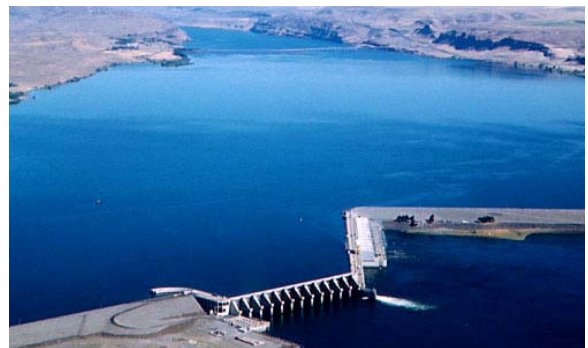
Wanapum Hydroelectric Development, Grant County PUD
