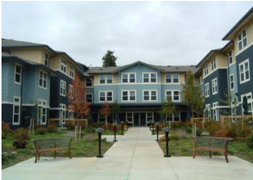
Angle Lake Court, King County Housing Authority
