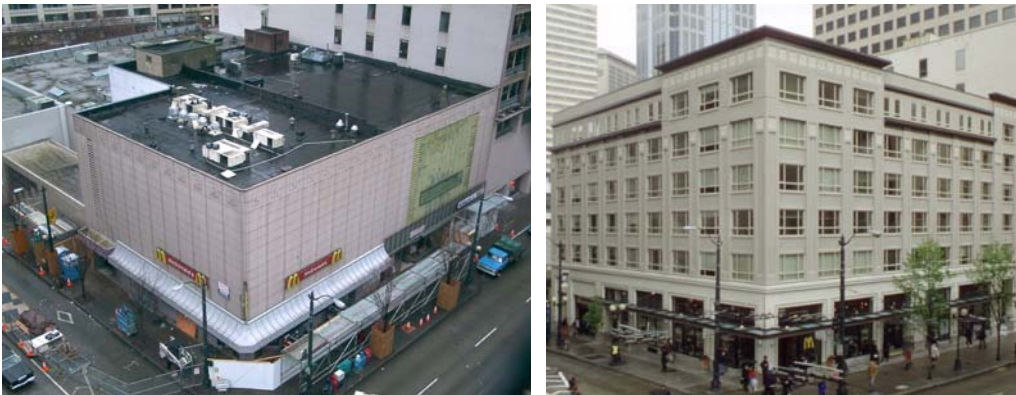
Housing Resources Group - The Gilmore Building before and after renovation, Seattle, Washington
