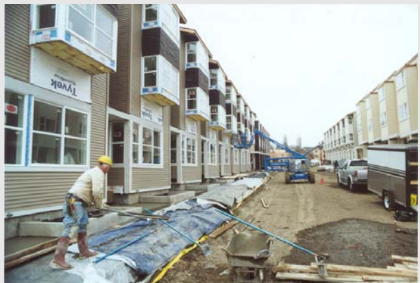
Seattle Housing Authority. Construction of NewHolly Phase II.
